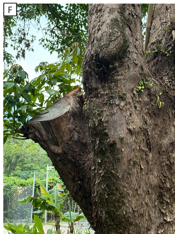
T71 ( Bischofia javanica ) Photograph showing the tree defect.
